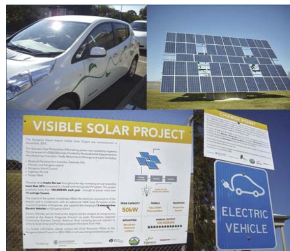
Kangaroo Island Visible Solar Project.
