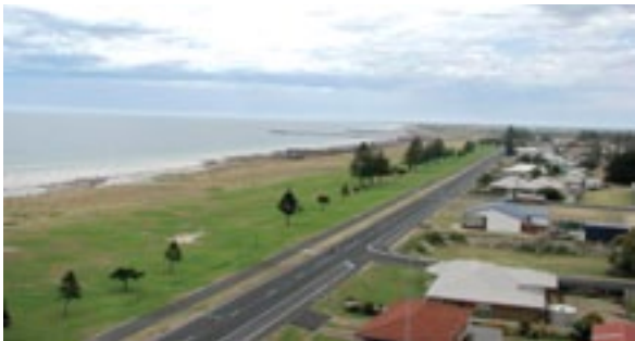
Section of Kingston SE foreshore area completely watered by recycled wastewater.
