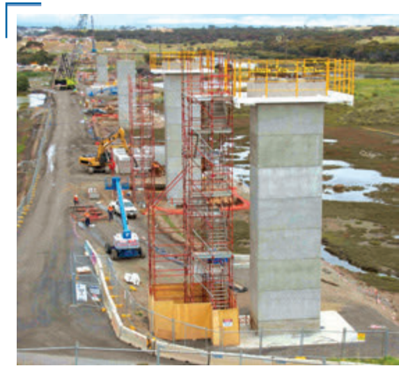
Seaford Rail Extension bridge spans across Onkaparinga River and tidal wetlands
