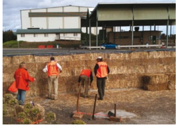
Straw bale wall under construction by volunteers
